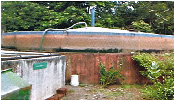
Nisargruna Biogas plant
