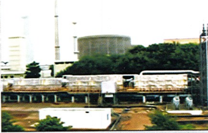
Desalination plant set up at Kalpakkam
